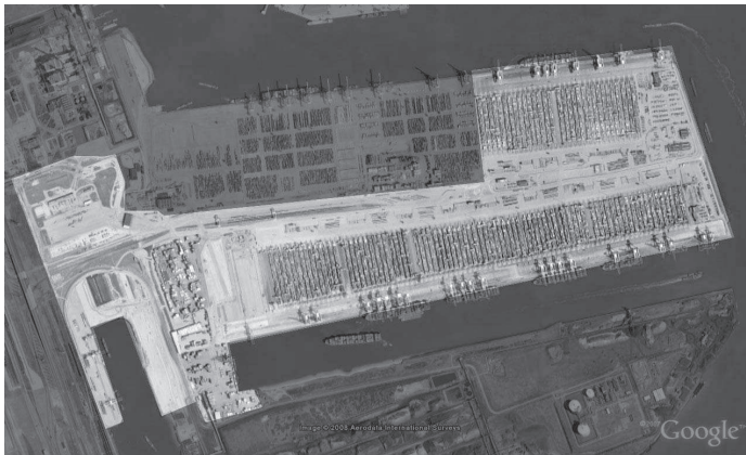
Figure 3.3: Aerial photograph of the ECT Delta terminal (Source: Google Earth©)
