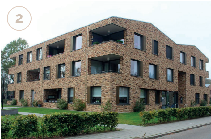
Residential care apartments, 3 stories (45 dwellings).
