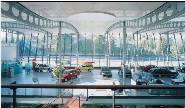
Figure 2.16 Roof structure with curved cellular beams
