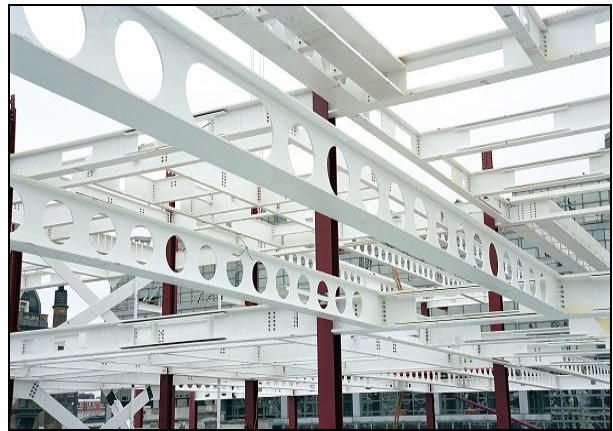
Figure 2.2 Various opening shapes in cellular floor beams
