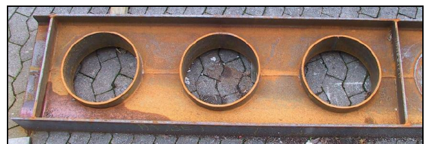
Figure 2.5 Circular reinforced openings
