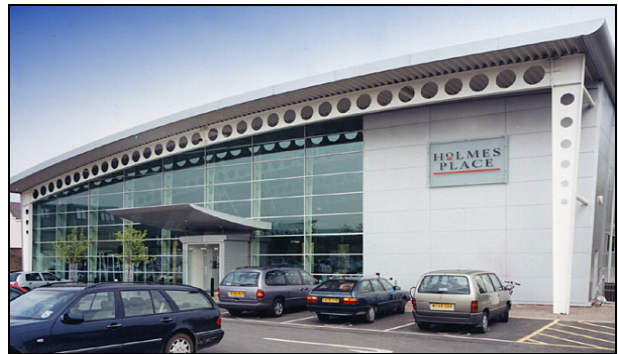
Figure 2.17 Cellular portal frame structure with tapered perforated columns
