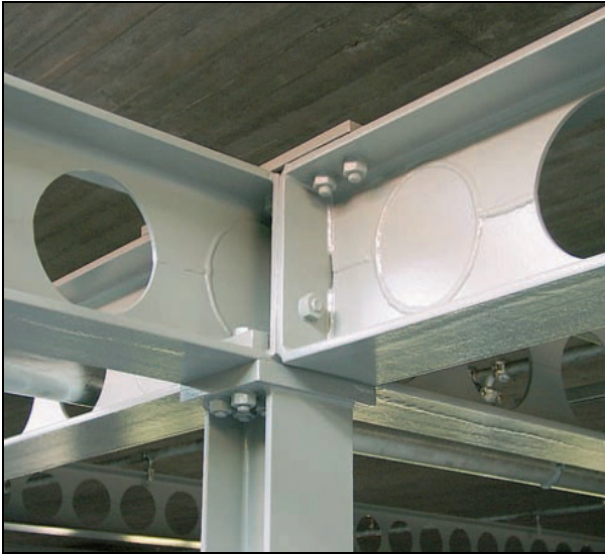
Figure 2.7 Filled web openings at support for increased shear resistance
