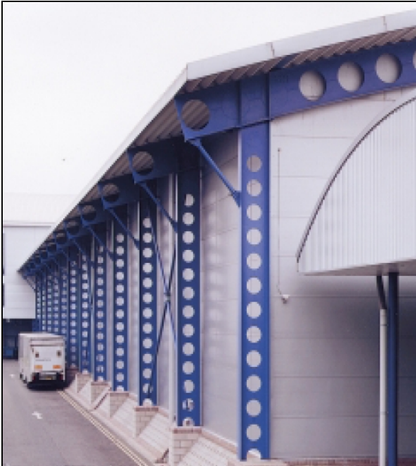
Figure 2.18 High-bay portal frame structure using cellular members
