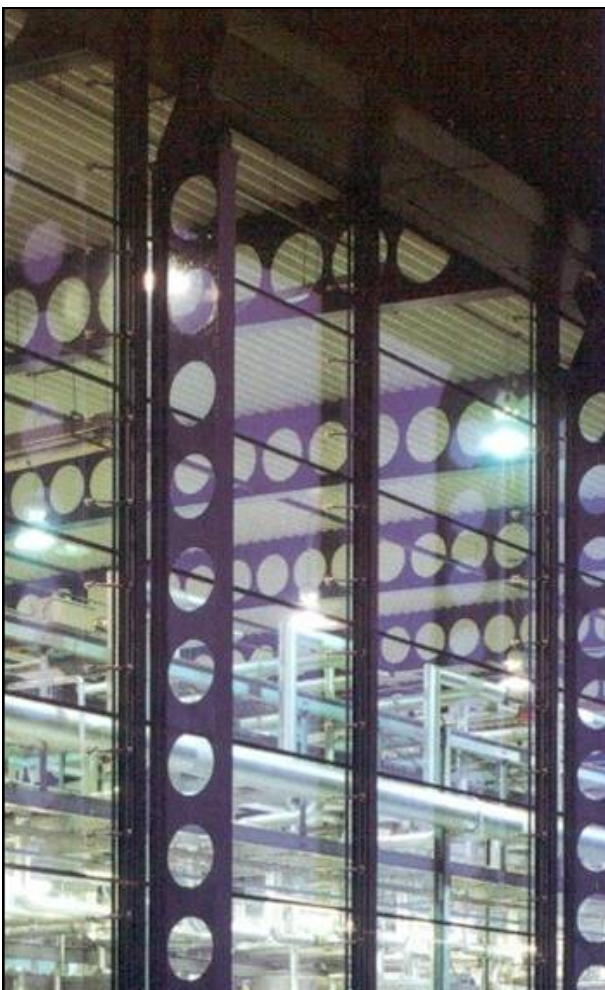
Figure 2.19 Cellular wind columns to support a glass façade
