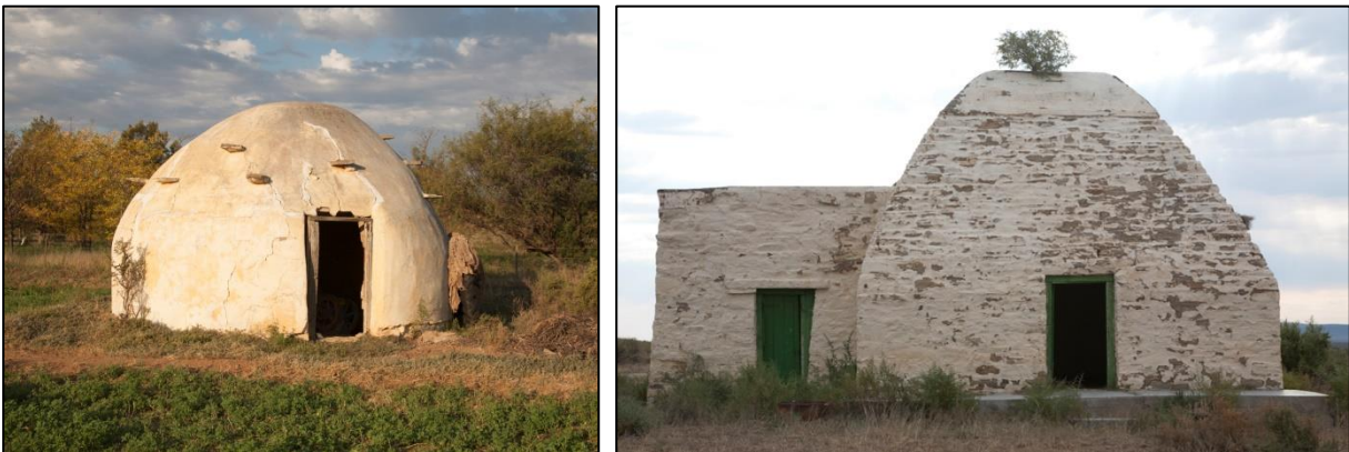
Figure 15.3: A small early corbelled house (likely 1820s or 1830s) may have originally been a kafhok, while a larger example has a square dome with a kitchen and wagon house added to the sides. Both are near Loxton.
