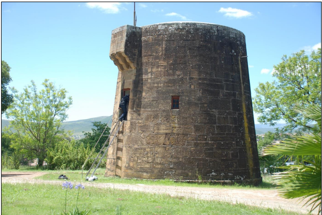
Figure 15.4: Martello Tower, Fort Beaufort.
