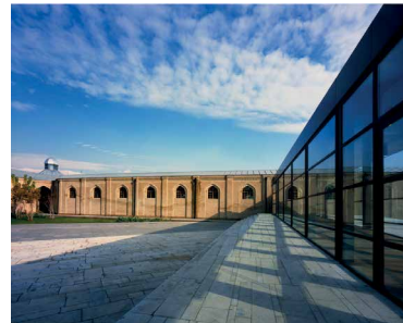
Qasr Garden Museum, after adaptive reuse (Ali Daghigh, https://rb.gy/nnoyvv )
