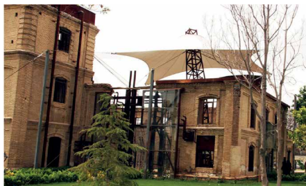
Textile museum, after adaptive reuse, with the addition of the tensile structure ( https://rb.gy/782mq )
