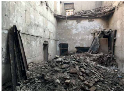
Argo Factory, before adaptive reuse (Shiar Studio, https://rb.gy/504bxi )
