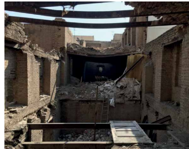
Argo Factory, before adaptive reuse (Shiar Studio, https://rb.gy/504bxi )
