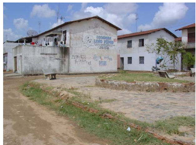
Photo 1.4. Example of derelict open public space in Fortaleza. Source: Rfurlani Architecture Office (2004).
