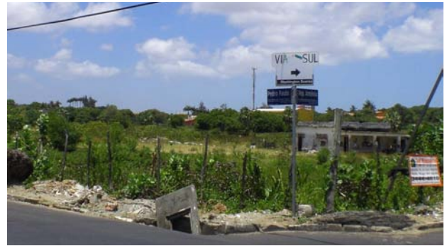
Photo 3.17. Derelict conditions of some sidewalks on the sub-centrality of Washington Soares. Source: Gilberto Studart.
