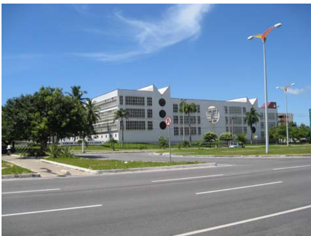
Photo 3.26. Location "I" - Relevant institutional buildings, such as the Forum of the city. Source: Author.
