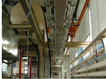
(b) Bottom view of the set-up. Left and right of the supporting steel beam, the tubes are mounted.
