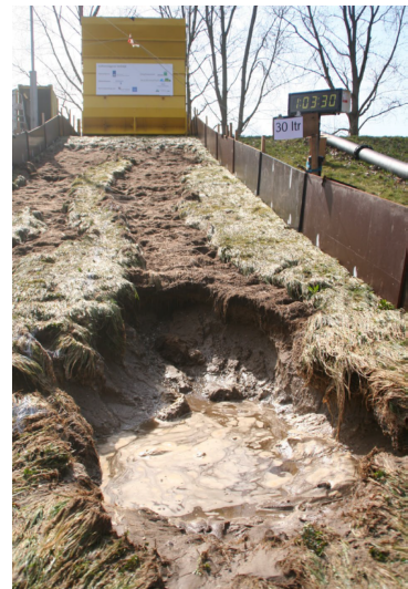
Figure 2.1: Example of dike failure due to overtopping with a simulator (EurOtop, 2018)
