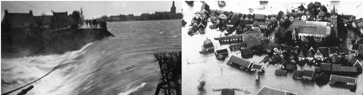
Figure 1.1: Dike breaching during the "Watersnoodramp" (Rijkswaterstaat, n.d.)
