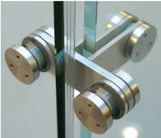
Figure 37: Bolted glass connection.
