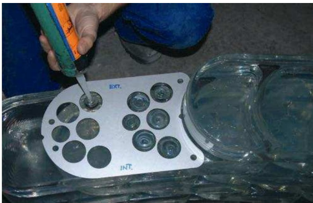
Figure 66: The distribution of adhesive on the glass blocks.
