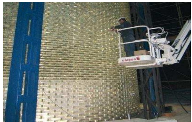
Figure 67: The process of the sealing.
