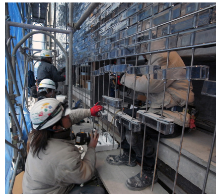
Figure 62: The assembly of the glass masonry.
