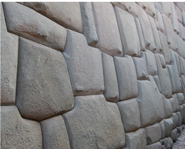
Figure 44 : Inca interlocking masonry walls.
