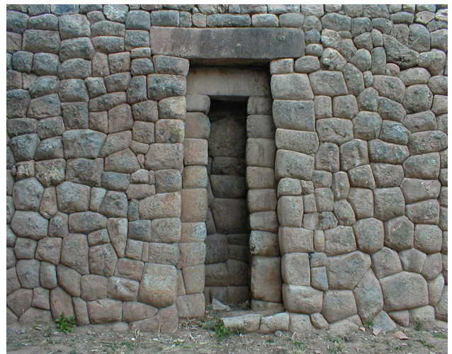
Figure 44 : Inca interlocking masonry walls.
