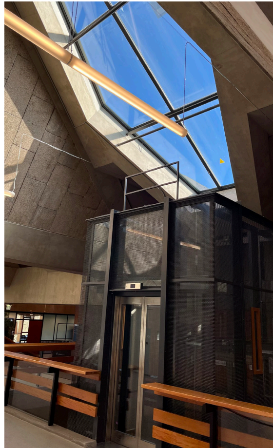
Fig 16. New elevator shaft by Mecanoo blocking one of six skylights in the foyer.
