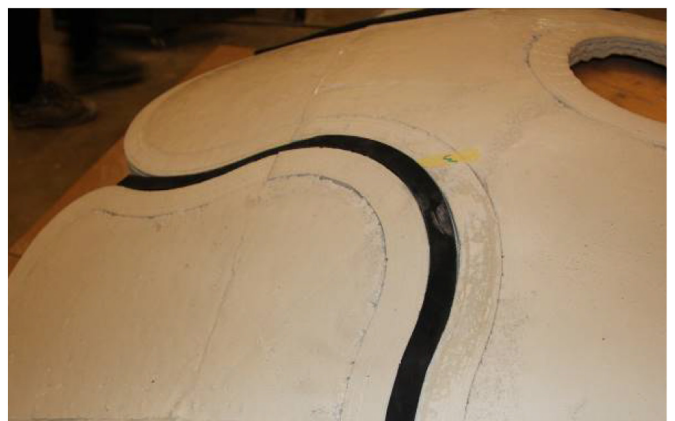
Fig. 23. Seam between two panels indicating a tight fit.
