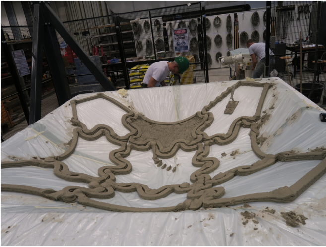
Fig. 18. Printing of first prototype.
