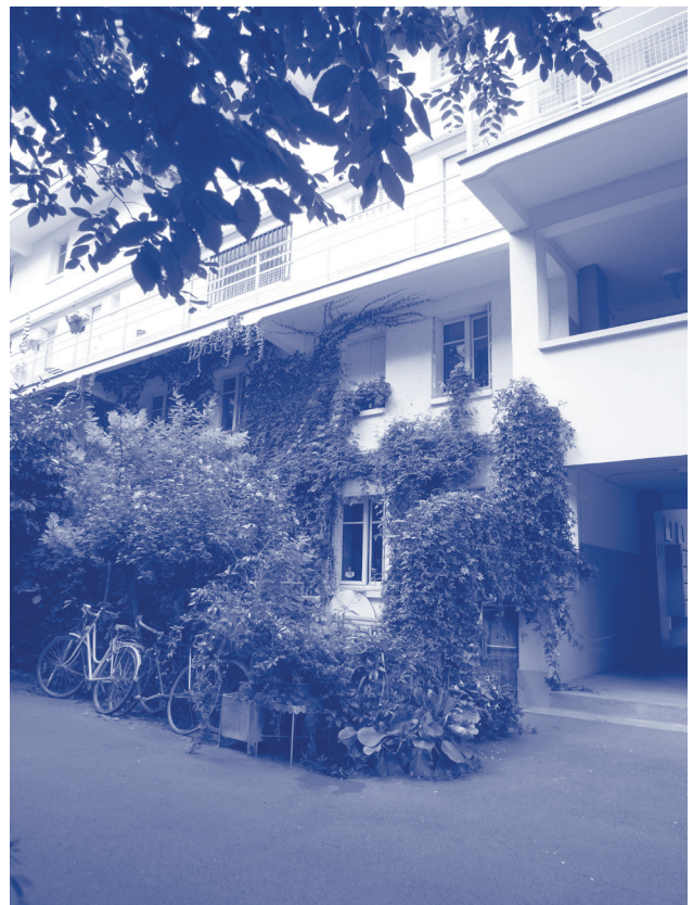
Figure 45 [Photo] Ground floor South side
