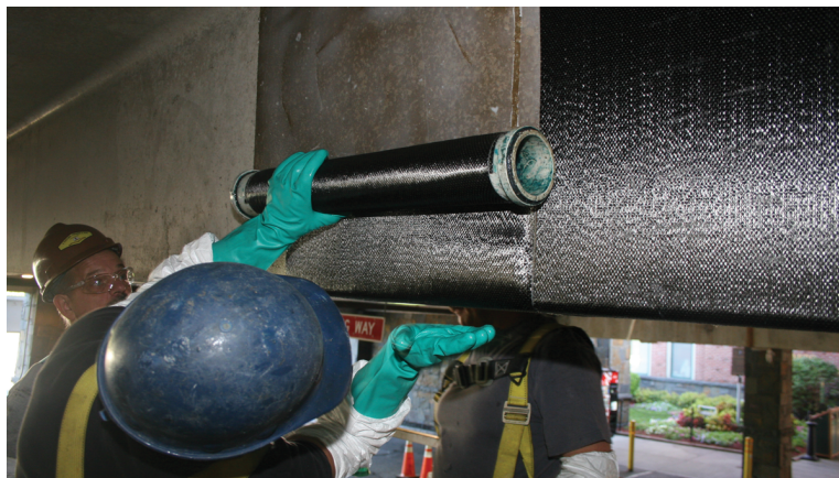
(a) Application of CFRP-wrapping.
