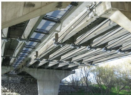
Figure 2.9: External prestressing tendons set-up as applied by Freyssinet [41].
