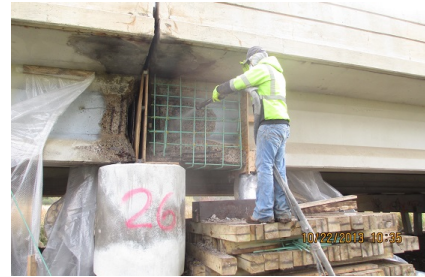
Figure 2.18: Application of UHPC strengthening [61].
