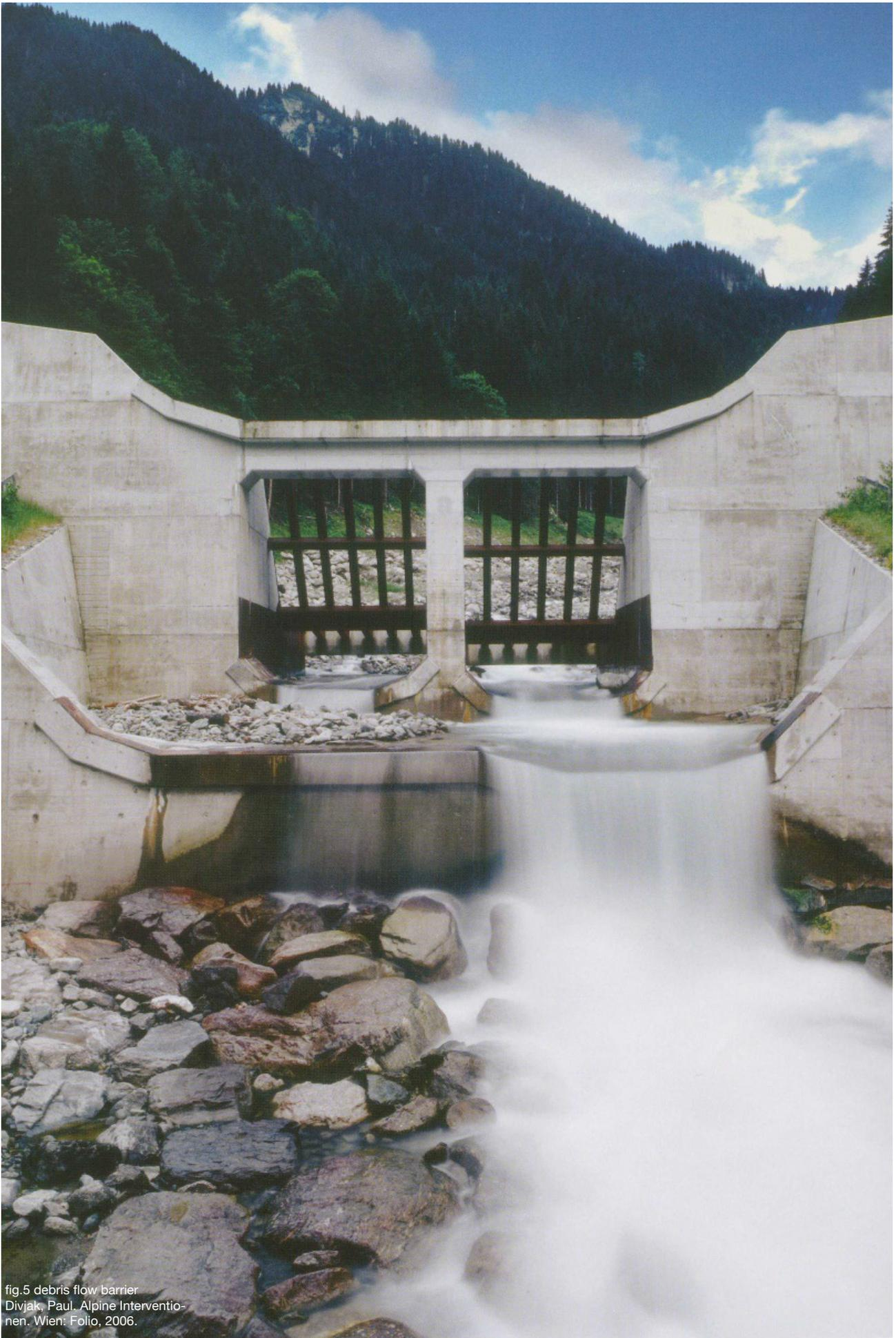
fig.5 debris flow barrier
