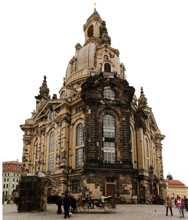
Figure 8. The north side and largest remaining original structure (dark stones) of the Frauenkirche. Retrieved from https://remotangles.com/2013/07/11/dresden-and-the-frauenkirche/
