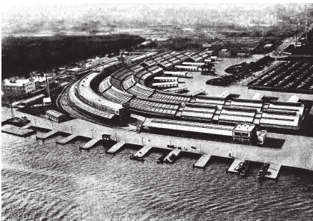
Figure 3 Aerial view of the Tsukiji fish market when it was finished in 1934. On the foreground were piers where seafood transported from Tokyo harbour off-loaded. Marine products traveled perpendicularly to the building's fan-shape, and entered Tokyo city. On the right the black rectangular shaped buildings are the outer retail market, which is still under operation today. Tokyo City. 1934. Aerial View of the Central Wholesale Market. Tokyo Central Wholesale Market Tsukiji Market - Architectural Drawings. https://ndlonline.ndl.go.jp/#!/detail/R300000001-I000000765120-00 .
