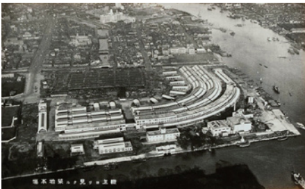
The fish market in Tsukiji, Tokyo. On the circumference aligned to a railway track (dismantled and replaced by an open air loading yard for freight trucks in 1987) is a steel structured shed where seafood trans shipped from the Tokyo harbour auctioned directly to wholesalers. The second and the largest part, sitting right next to the auction space, is a wholesale market, in which marine products are further sorted, graded and sold to retailers and restaurants from the entire metropolitan area. At the center point of the market are 8 loading sheds that further distribute the fish to the city.
