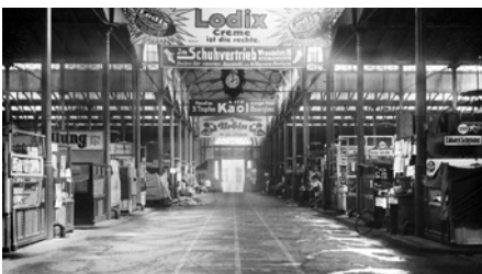
Photo of Markthalle IX (now Markthalle Neun). As part of the schematic plan to build a new food supply chain that met the need for a modern metropolitan, the Markthalle IX followed the same architectural logic of a steel structure roof, efficient drainage system and natural lighting, providing Berliners a comfortable and hygienic food shopping place. Source: markthalleneun.de/ueber-uns/geschichte/
