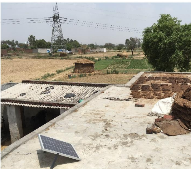
Image 5 : A solar panel installed on the roof of rural household.
