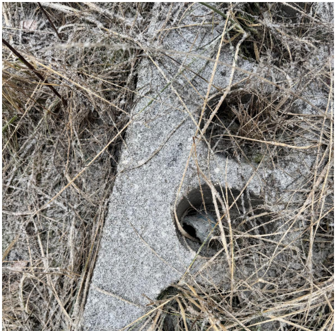
Figure 25 | Concrete blocks for heavy machinery
