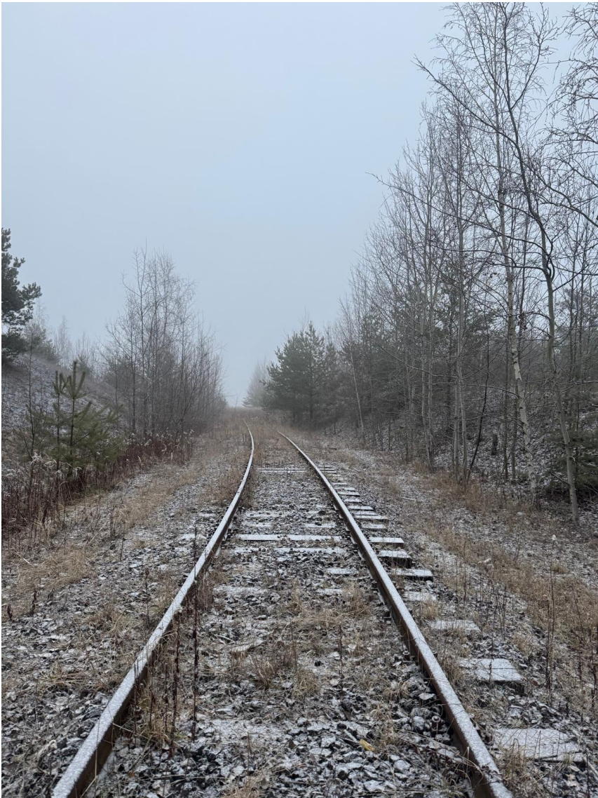
Figure 24 | Old railway structure on the Makoszowy Heap
