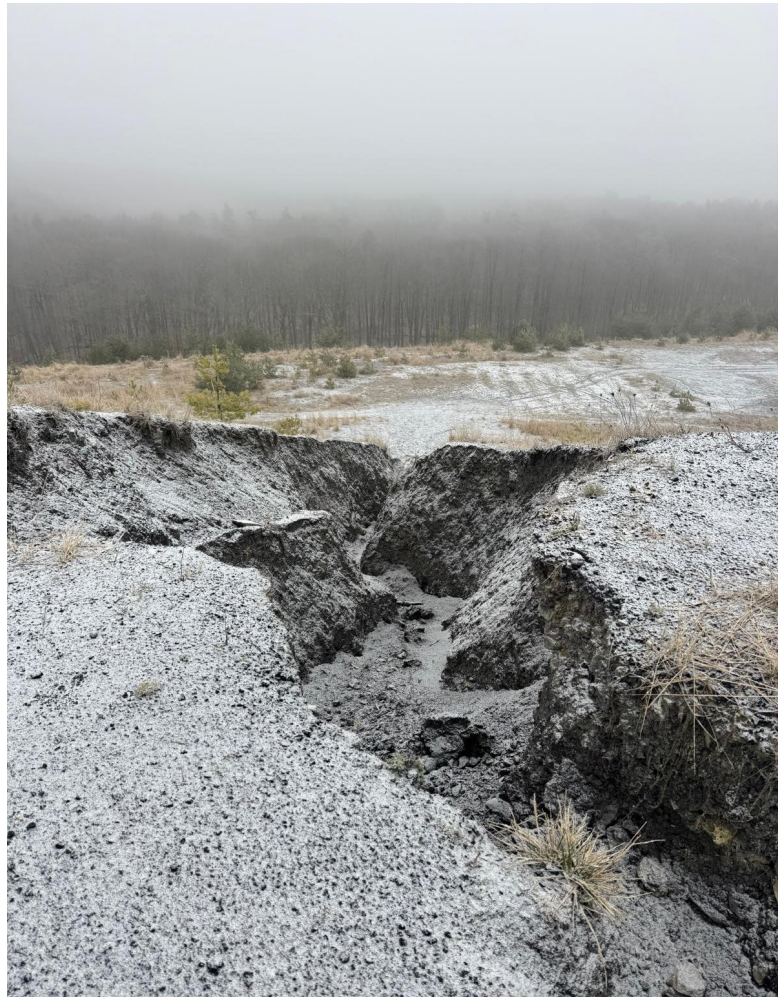
Figure 1 | Erosion crack on the heap
