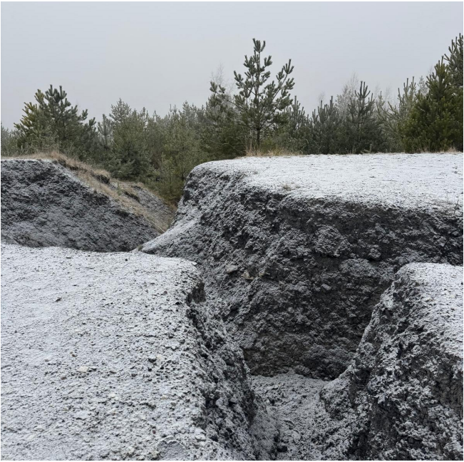
Figure 23 | Small erosion crack measuring approximately 2m in width and 10m in length
