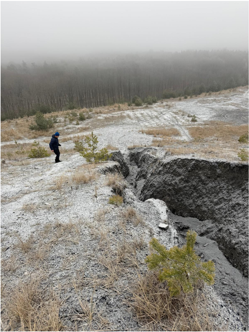
Figure 22 | Erosion crack measuring approximately 5 m in width and 50 m in length
