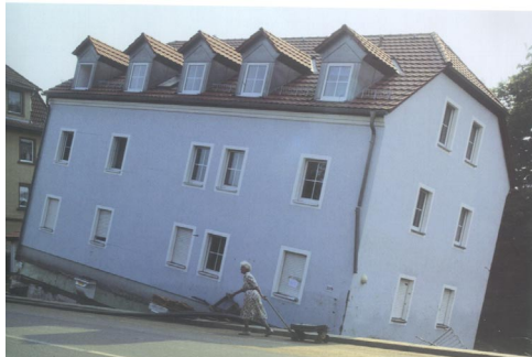
Photo 2 Scour of the foundation during the flood in August 2002 in Germany(Reimer, 2002)
