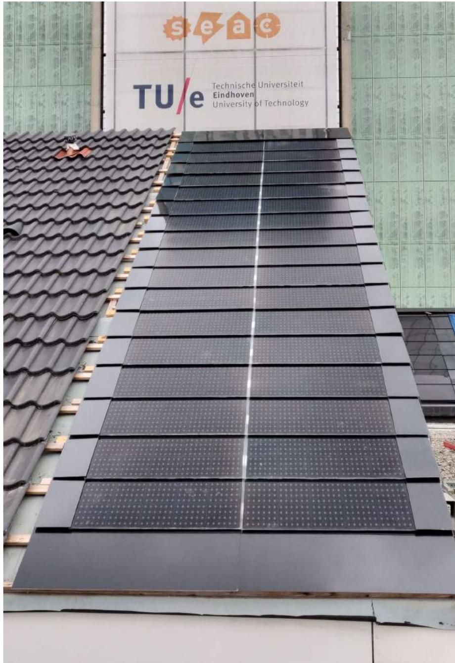
**Figure 4.11:** Completed BIPVT setup
