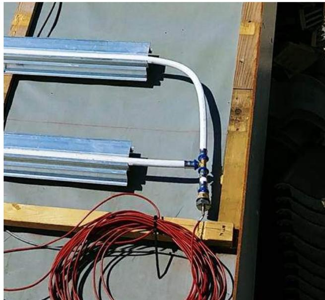
**Figure 4.5:** PT100 temperature sensor placement along the fluid flow
