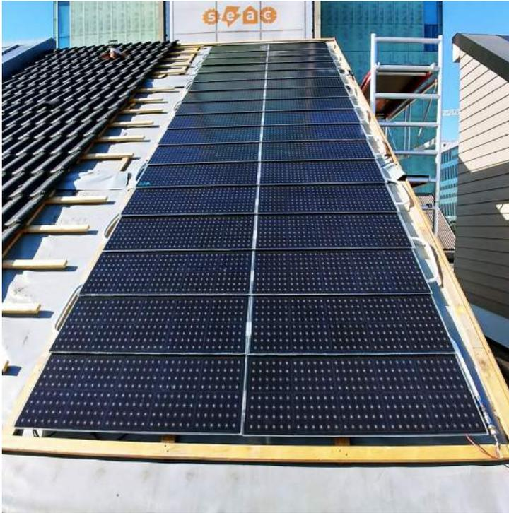
(a) Solar panels installed atop the dummy roof
