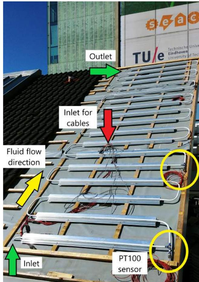
**Figure 4.8:** Mounting structures and pipes atop the dummy roof
