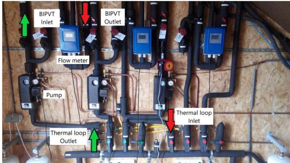
**Figure 4.6:** Thermal fluid framework under the dummy roof
