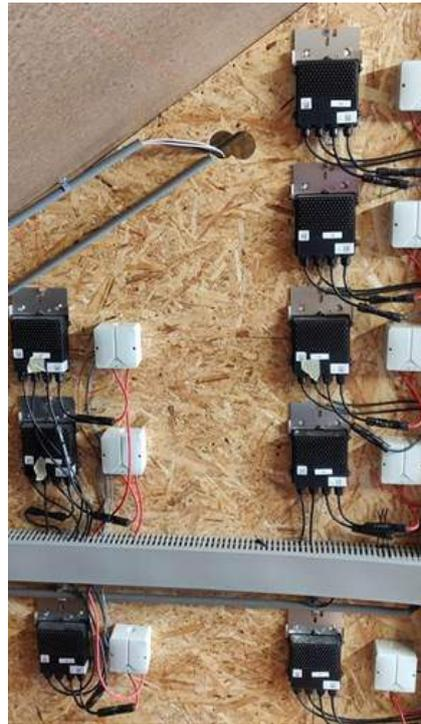
(b) Power Optimiser/Charge controller connections inside the dummy building
