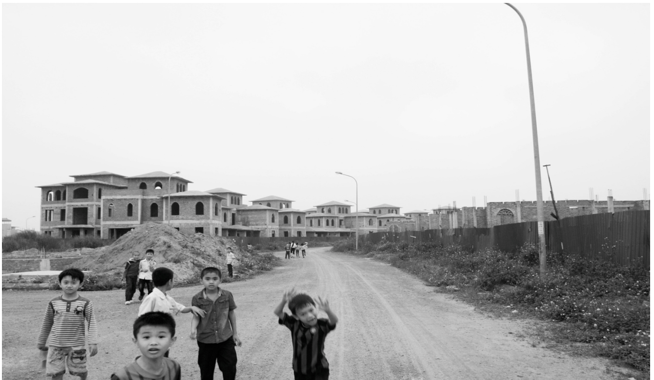
Figure 3. Nam An Khanh: South view of current situation (photo by W. van Faassen, 2013).
