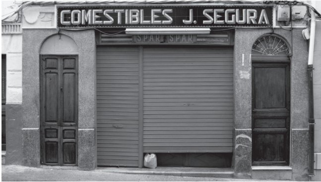
Fig. 1. Functional integration. Adopted several decades ago, metal shutters are part of a consolidated landscape. While their owners cannot do without them, for others, these are controversial because they disfigure the historical environment's integrity. Image: Juan A. García-Esparza, 2019. Chair of Historical Centres and Cultural Routes, Spain
