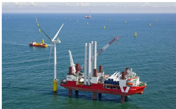
Figure 2.2: MPI Resolution installing wind turbines [18]
