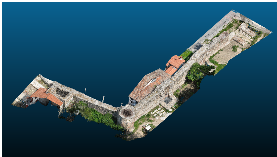
Figure 5.4: East side of the Byzantine Wall in CloudCompare
