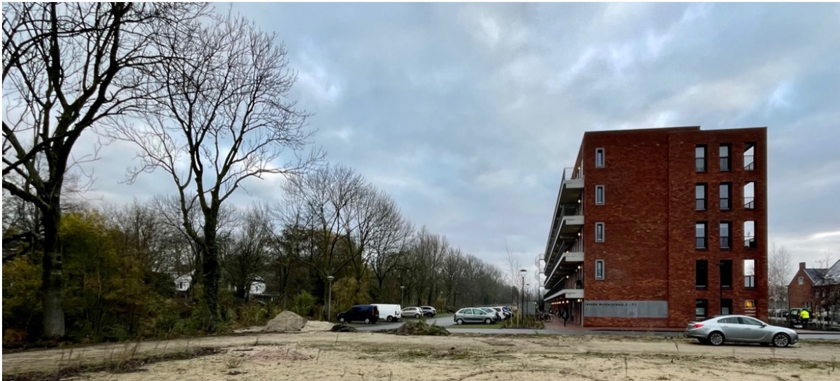
Figure 14: Low-rise residential building, left the Professor Evertslaan, Delft (own image, 2021)
