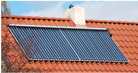
Figure 11: A solar boiler on a rooftop
