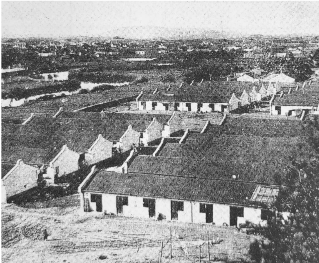
Figure 18: Different from the garden-style layout of employee housing, civilian housing adopts a row-type layout, and the living units are simpler. Source: Capital Design Technical Commission Office. The City Plan Of Nanking , 204.
