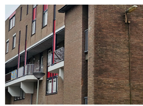
Red Trespa panels from facade
