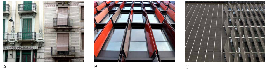
FIG. 3.1 Evolution of adaptive façade components from manual towards intelligent. The evolution is exemplarily shown by shading devices: (A) traditional shutters (building from 19 th century) (Image by author), (B) automated shading elements of oval office by Sauerbruch & Hutton, Colonia (DE) (Image licensed under CCO Public Domain), (C) intelligent kinetic skin of ThyssenKrupp Q1 Headquarter by JSWD Architekten and Chaix & Morel et Associés, Essen (DE) (Image courtesy of Günter Richard Wett).
