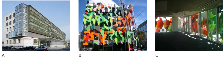
FIG. 3.7 Examples for static constructions providing passive adaptation. (A) Energybase office building in Vienna (AT) by pos architekten, 2011: the folded south façade prevents in summer direct solar gains and allows at the same time maximum PV electricity production (Image courtesy of Hertha Hurnaus in 'nachhaltig wirtschaften, 2018'). (B and C) Pixel office building in Melbourne (AU) by studio505: the fixed shading system is parametrically designed solution, optimized by dynamic daylight and thermal simulation assessments (Image by author).
