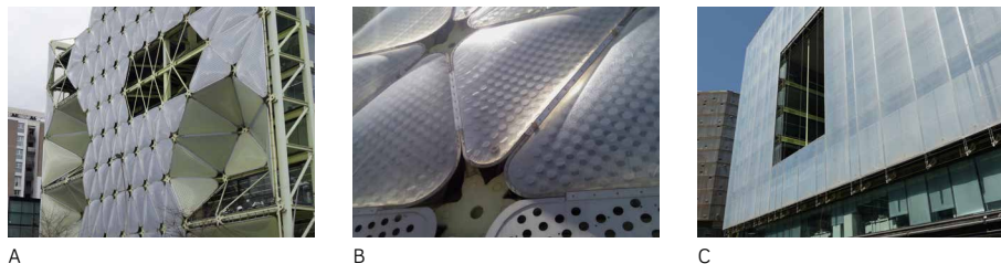
FIG. 3.5 Example for embedded adaptive materials. (A and B) South-east façade of the Media TIC Building in Barcelona (ES) by Cloud 9: the layers of the triangular ETFE membranes are pneumatic and can modify the light transmission by changing the spacing of the patterned layers (Image courtesy of Ulrich Knaack). (C) The south-west façade of the same building is using a different approach to light selection by changing the air density of the gas in the cushions, which creates a solar filter (Image by ACME, 2018).
