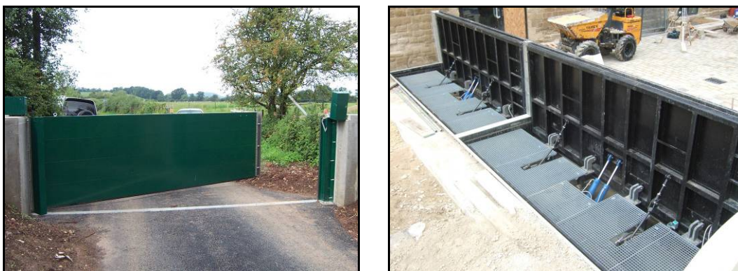
Figure 5.11 Fully preinstalled flood gates
