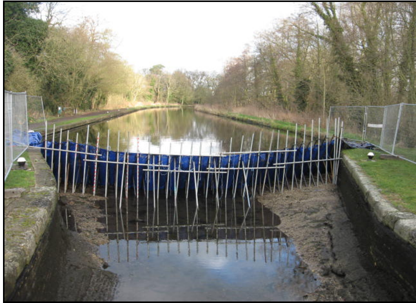
Figure 5.6b Flexible frame barrier in operation
