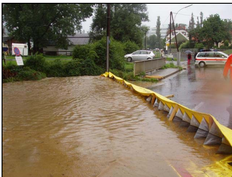
Figure 5.5b Flexible free-standing barrier in operation
