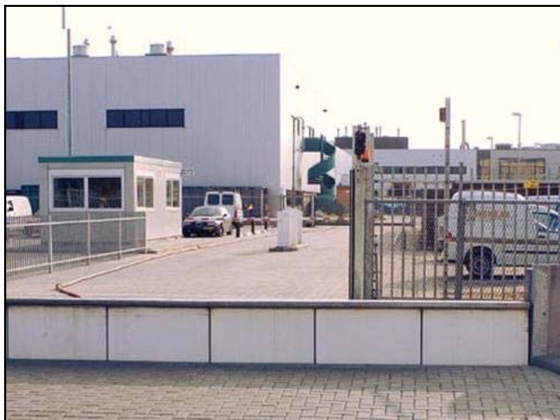
Figure 5.10c Automatic sectional barrier
