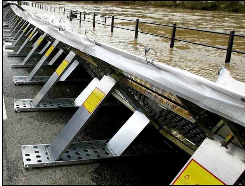
Figure 5.6c Rigid frame barrier in operation
