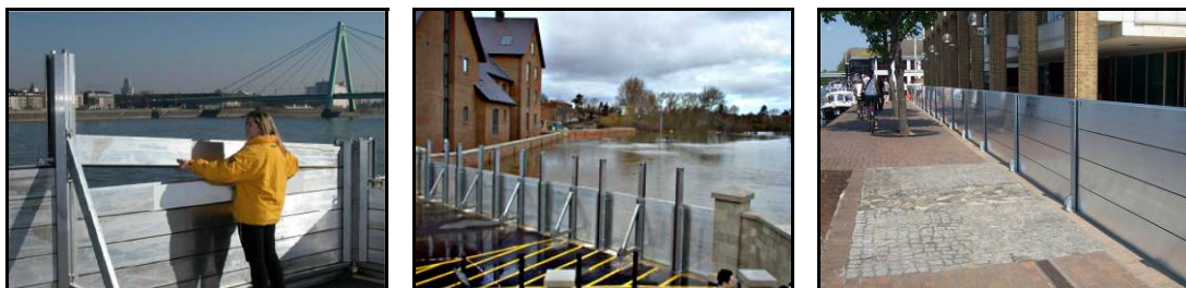
Figure 5.9c Demountable frame barriers
