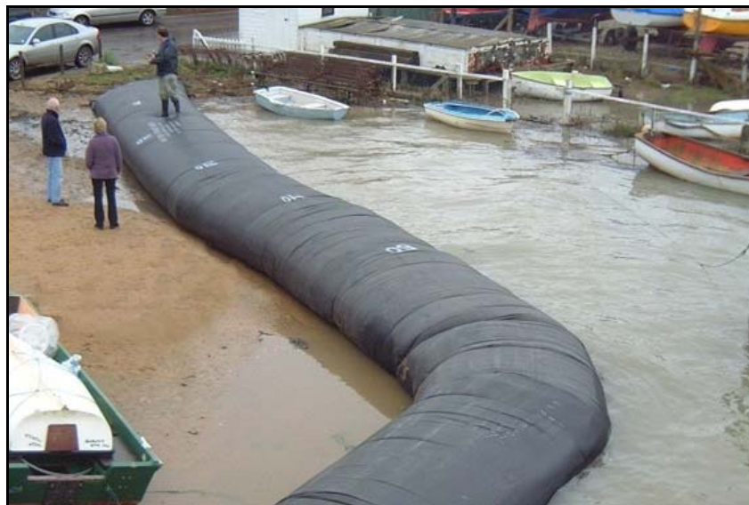
Figure 5.3c Water filled tube in operation
