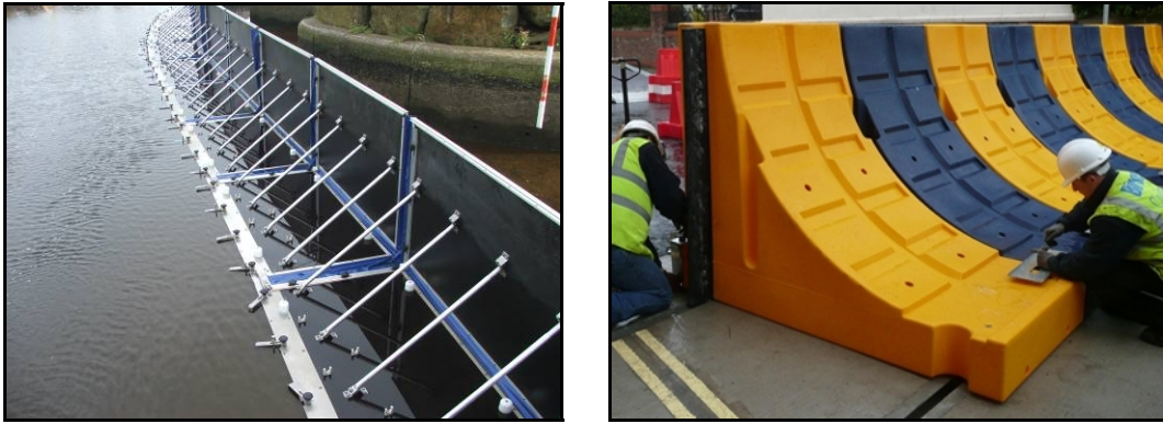
Figure 5.8d Rigid demountable free-standing barriers
