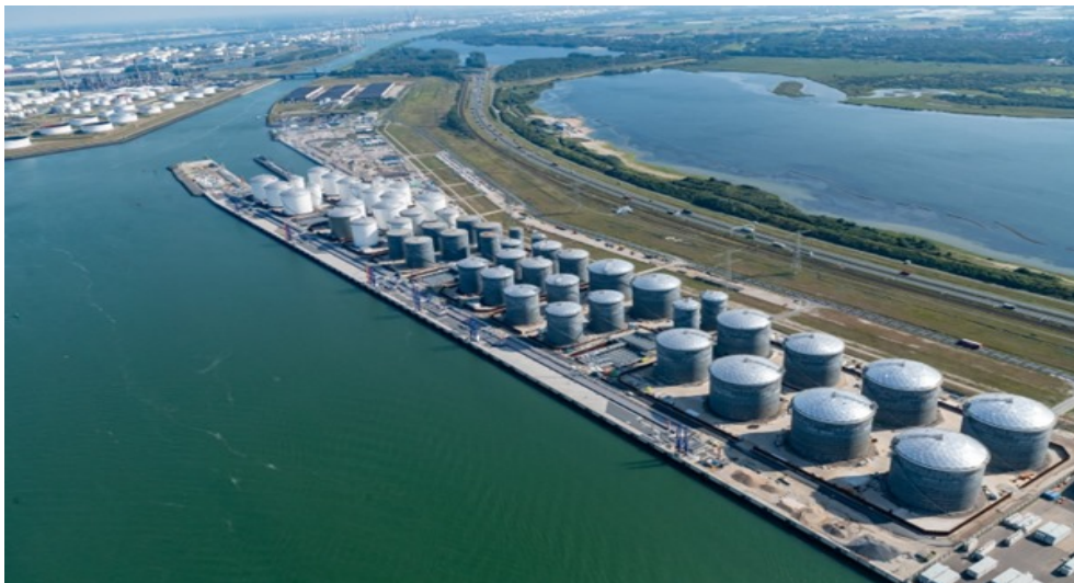
Figure 3.1: HTT Quay wall after the construction of storage tanks enclosed within bund walls
