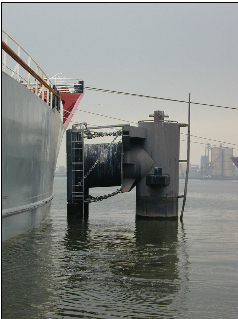
Figure 2-6 Ship mooring to a flexible dolphin fitted with a fender
