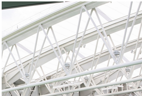
Figure 2.25: Wimbledon roof truss bolted joint.
