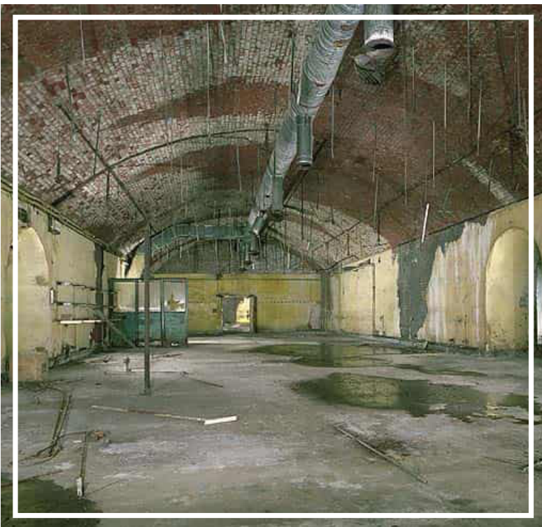
Staff mess room at west side of site
