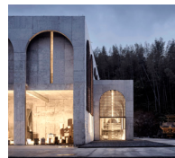
BingQing Wood Kin Factory, A2L architects
