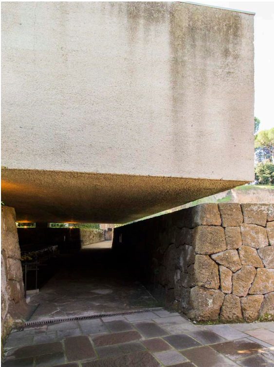
Fosse Ardeatine Mausoleum, Mario Fiorentino and Giuseppe Perugini Sprayed concrete
