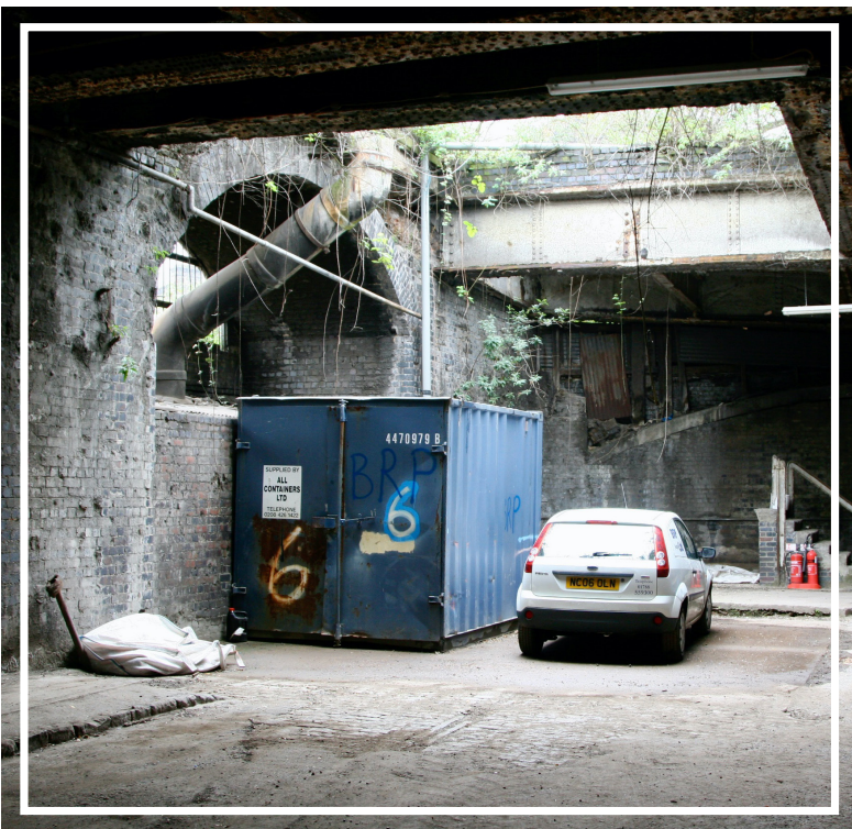
Pit for hydraulic wagon lift on south west of site
