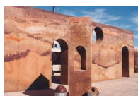
Cast earth construction, Heriberto Zapata
