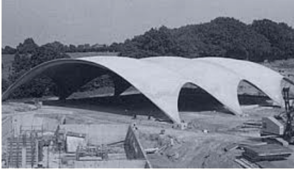
Figure 4.1 (left) The construction of Isler shells in Norwich Sports Park, Norwich England, 1991. (right) Physical model made by Isler.
