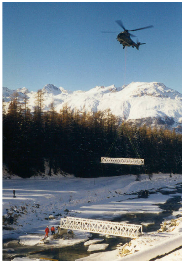
Figure 1.6 Temporary lightweight pedestrian bridge in Pontresina (Switzerland), installed each fall and removed in the spring (1997) [16].
