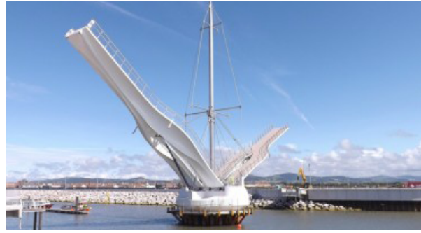
Figure 1.5 (left) Pont y Ddraig, or Dragon Bridge, at Sandown, Isle of Wight, UK. (right) FRP decks for Pont y Ddraig under construction at AM Structures, Sandown, Isle of Wight [14].
