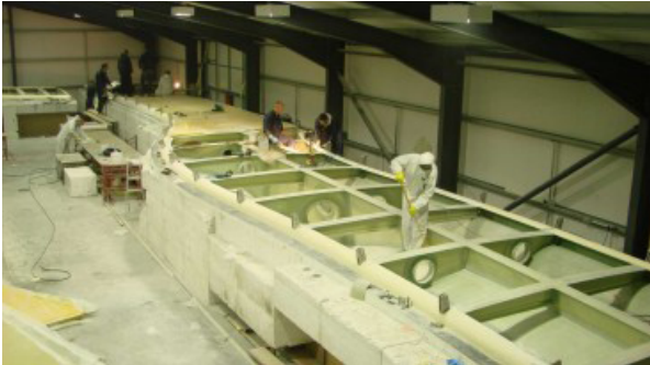
Figure 1.5 (left) Pont y Ddraig, or Dragon Bridge, at Sandown, Isle of Wight, UK. (right) FRP decks for Pont y Ddraig under construction at AM Structures, Sandown, Isle of Wight [14].
