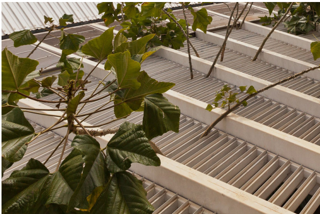
sun protection louver in polycarbonate
