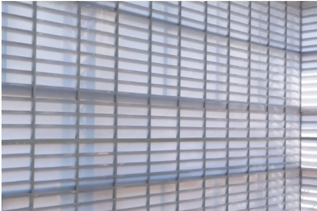
polycarbonate louvers “comovent” type
