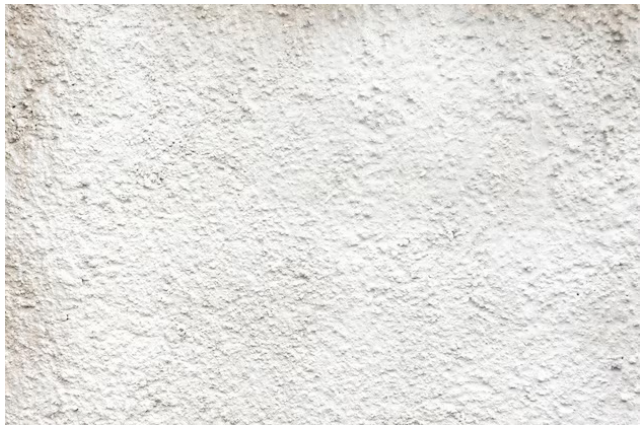
renovation of texturized plaster painted white
