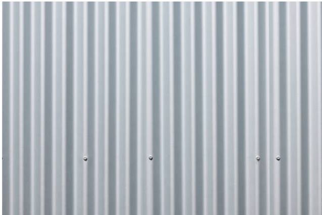
moving panels in corrugated zync sheets
