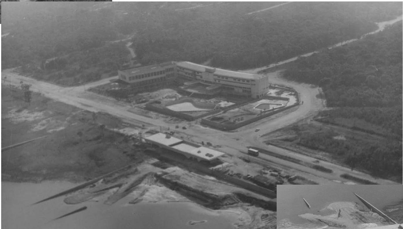
the club under construction, early 1960s
