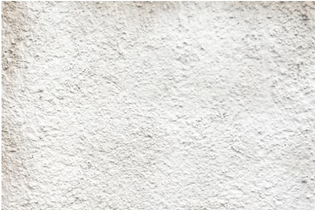
renovation of texturized plaster painted white
