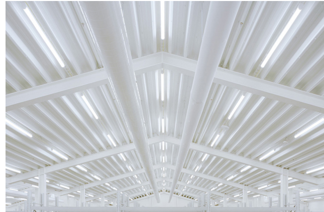
renovation of texturized plaster painted white
