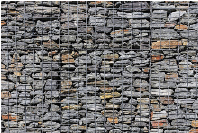
gabion retaining wall
