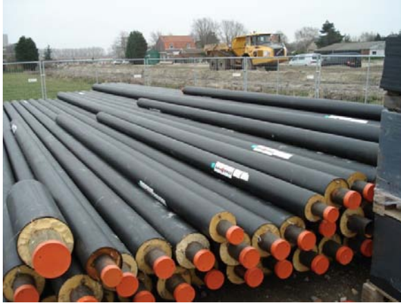
Figure 08 district heating pipes for the Harnaschpolder in Delft. 22
