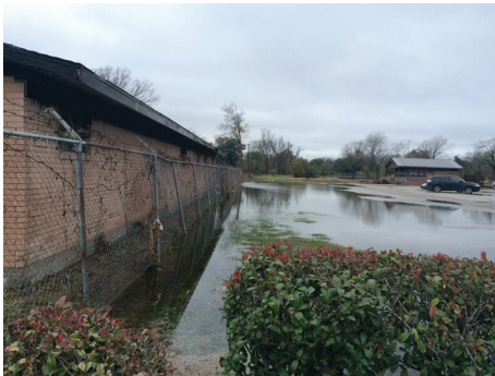
Flooding during heavy raining day
