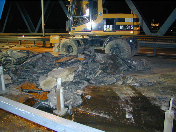
Figure 6-56: Removing asphalt
