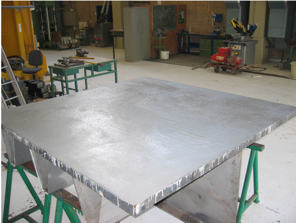
Figure 6-30: Test panel A with RHPC surfacing directly after power floating
