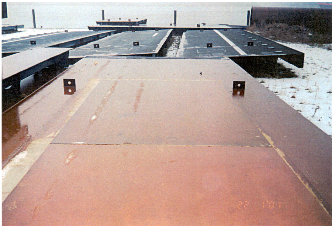
Figure 7-8: Application test bonded second steel plate
