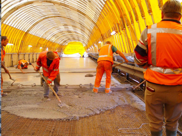
Figure 6-68: Casting concrete
