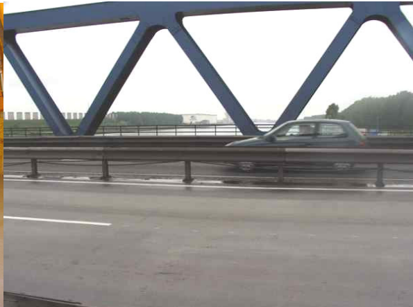
Figure 6-70: Finished RHPC surfacing
