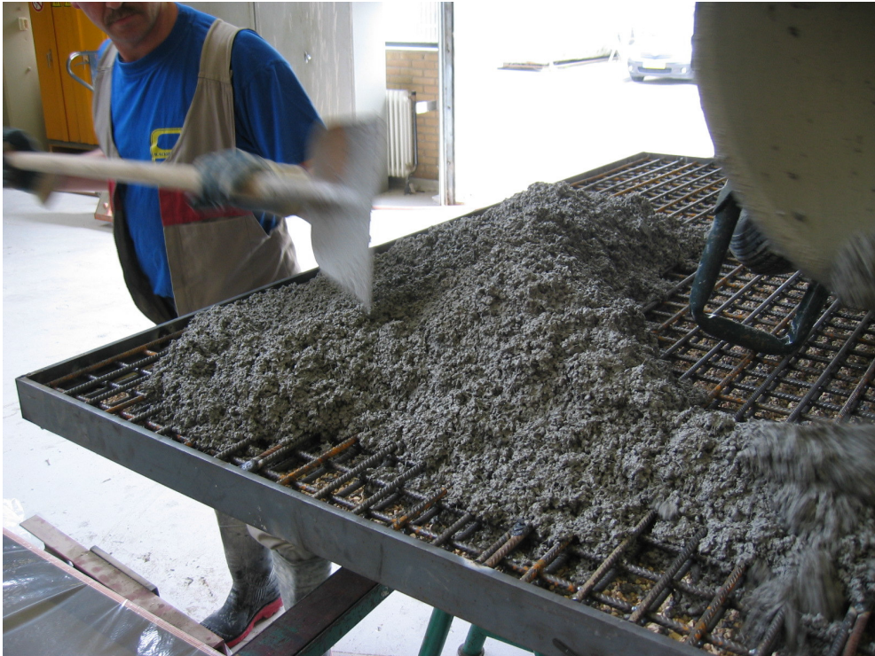
Figure 6-29: Mesh reinforcement & casting RHPC on test panel A
