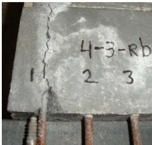
Figure 7-60: Splice failure of ribbed steel bar in C100, 3 mm concrete cover
