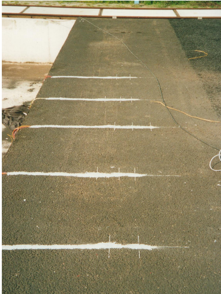
Figure 4-59: Connecting cables with protection on top of the surfacing
