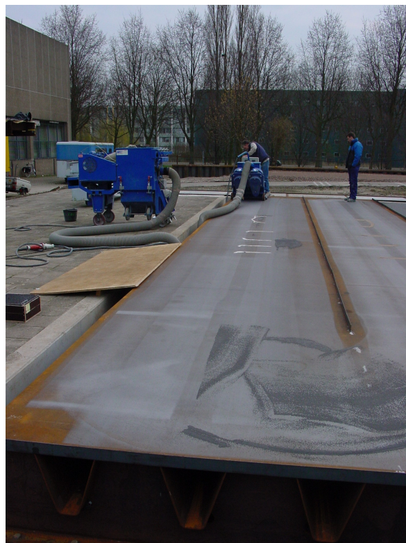
Figure 4-49: Shot blasting deck plate before application surfacing
