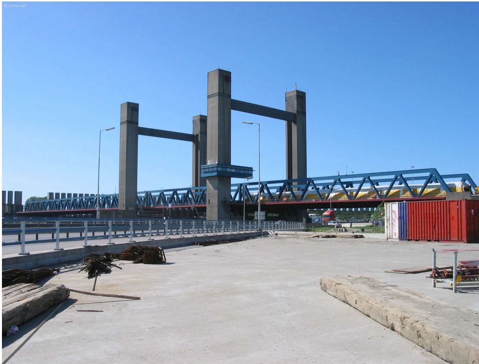
Figure 6-54: Caland Bridge in the harbour area of Rotterdam
