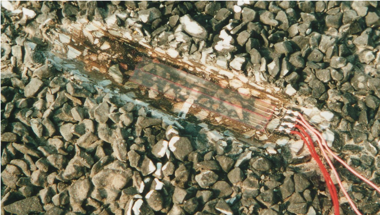
Figure 4-57: Strain gauges on top of mastic asphalt surfacing (duplicated gauges)
