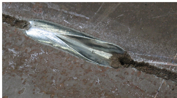
Figure 5-8: Burn through due to excess weld energy
