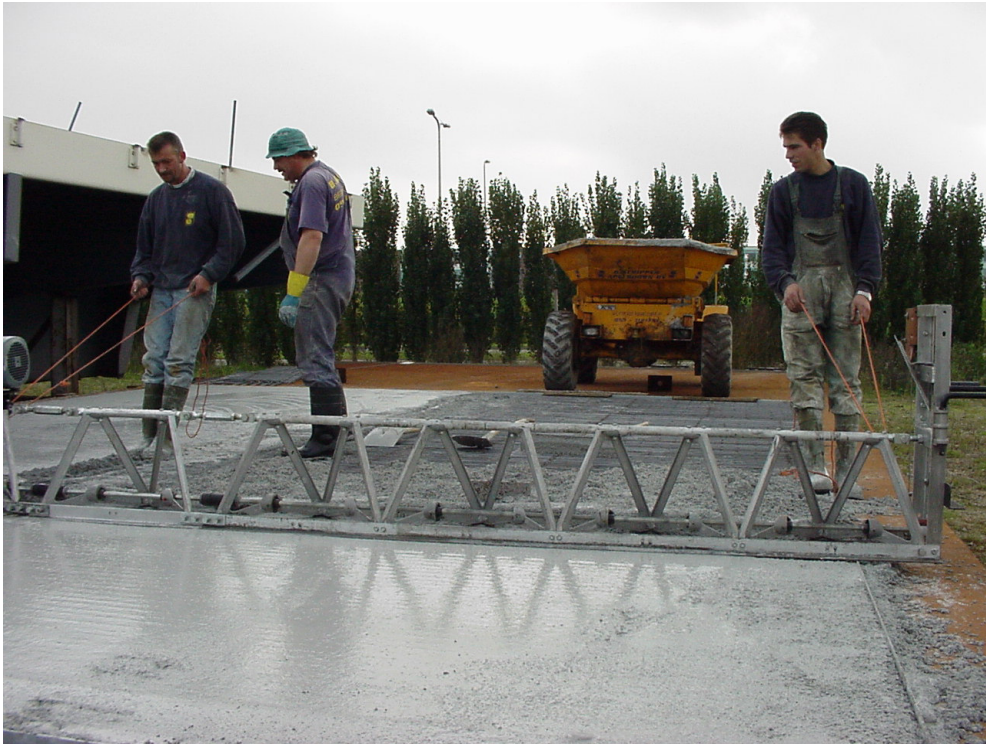
Figure 6-19: Compacting with vibrating screed on test area 1
