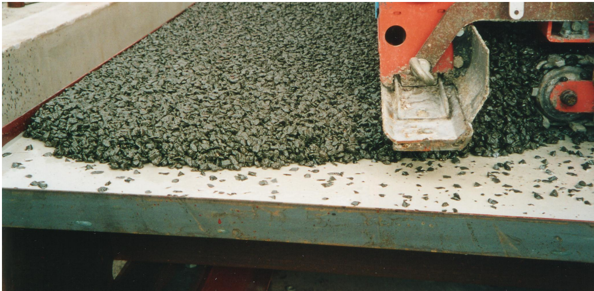
Figure 4-52: Application ZOK surfacing of 50 mm
