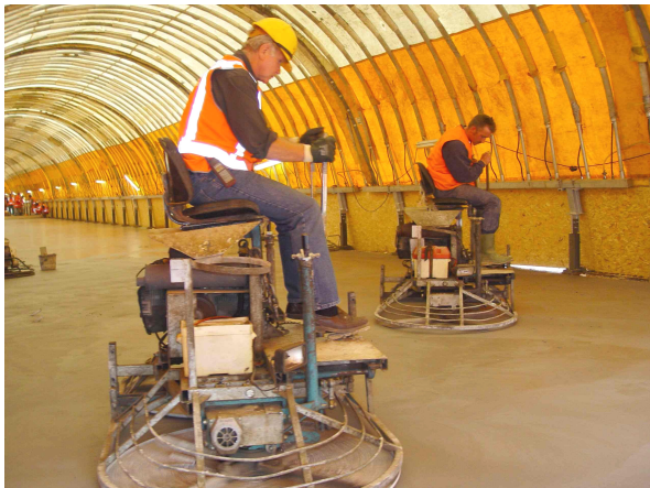
Figure 6-69: Power floating
