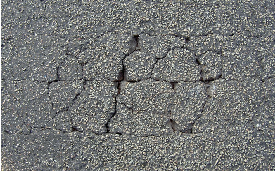
Figure 2-14: Visual observations possibly indicating deck plate crack
