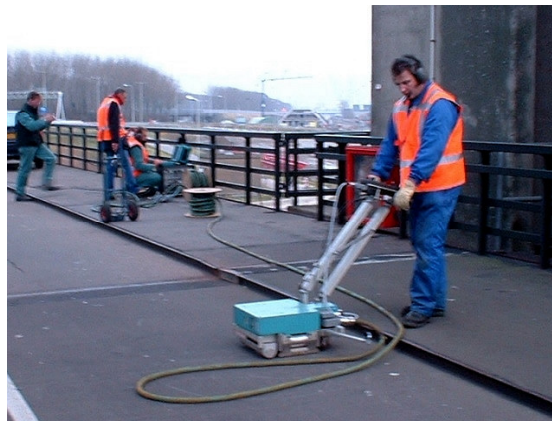
Figure 8-12: SLOFEC inspection being carried out on Caland Bridge
