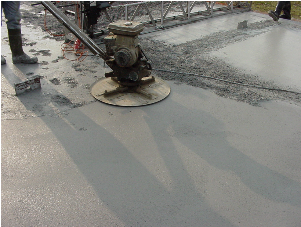
Figure 6-20: Power floating surface on test area 1
