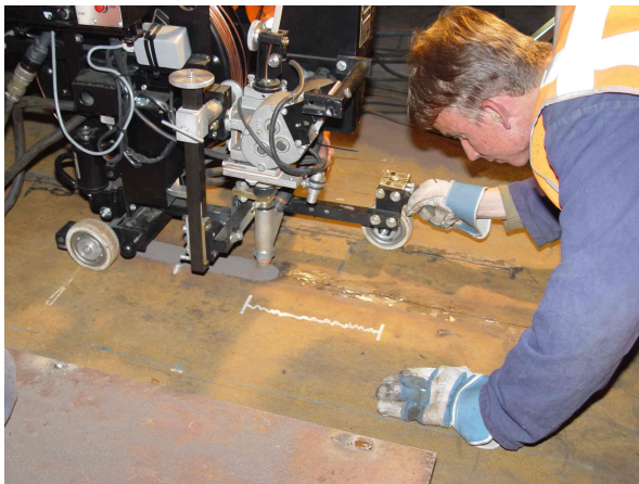
Figure 6-61: Submerged arc welding
