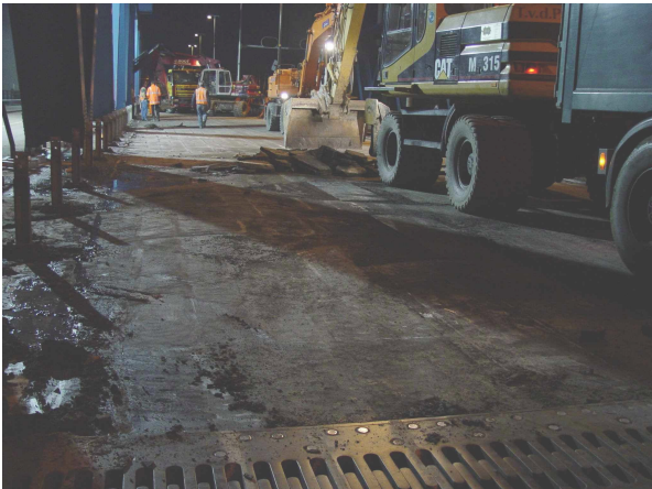
Figure 6-57: Removing asphalt
