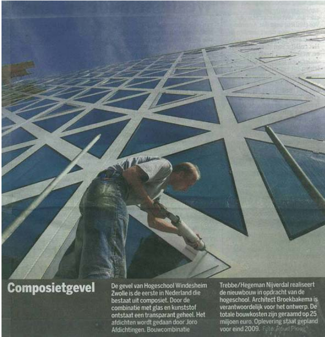
Installation of GRP facade in Windesheim, Zwolle. (source: http://www.trebbe.nl/actueel.aspx?id=160&archief=2009 )
