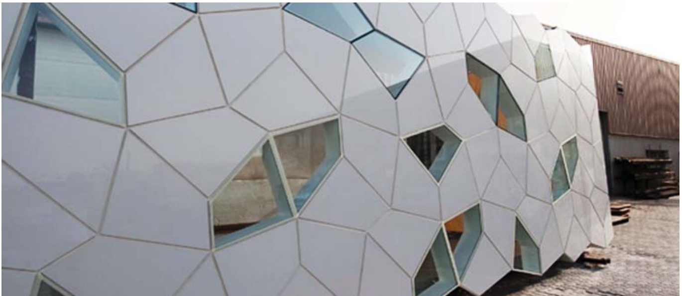
GRP facade element for RAK Gateway. The prototype panel built by PCT, measures 8x4m and is one of the approximately 1000 required to clad the entire building. (source: http://www.pct.ae/composites_projects.php?project=18 )
