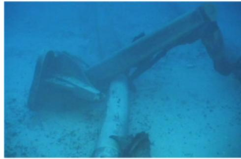
Figure 2.3: Trapped anchor at Transmediterranean Pipeline System [5]
