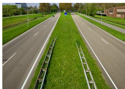
Figure 2-3 Rural distributor road type I
