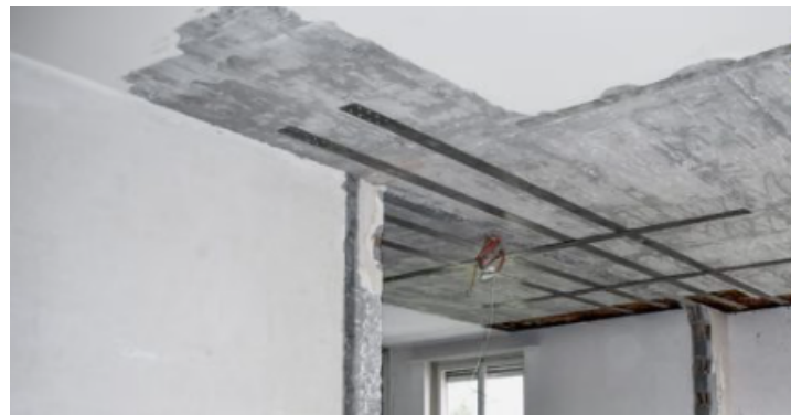
Figure 7.6: Example of memory steel used to strengthen a concrete floor(re-fer AG, 2021)
