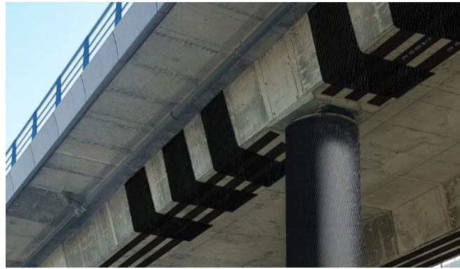
Figure 7.5: Example of CFRP lamellas used to strengthen a concrete bridge (Simpson Strong-Tie, 2024)
