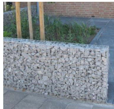
Figure 25: gabion example (bigbagsiergrind.nl, n.d.)
