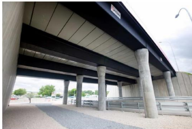
Figure 52 M111 Bridge (MARA, 2015)
