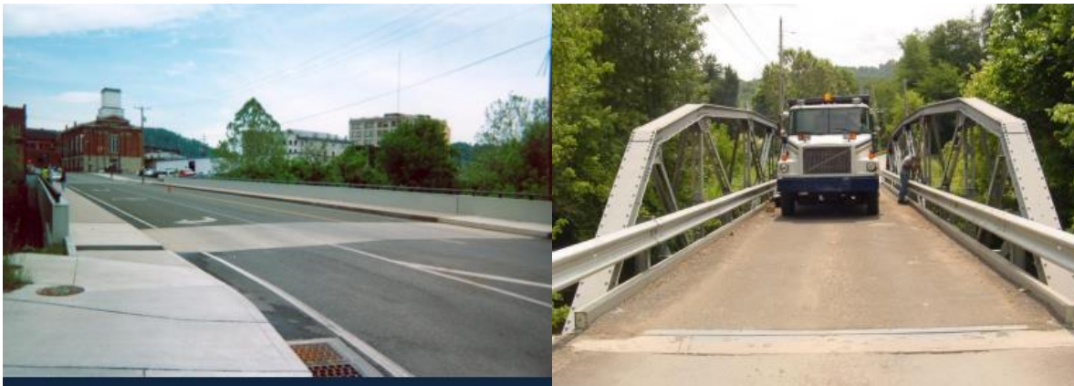
Figure 48 Market street bridge and katy truss bridge(GangaRao,2012)
