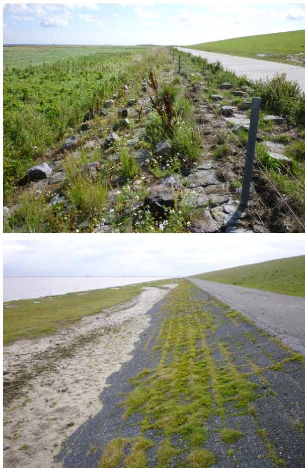
Figure 2: Dike with an adjacent broad salt-marsh zone (Elisabethgroden, Germany, top) and dike with a narrow salt-marsh zone (Dollard, Netherlands, bottom).
