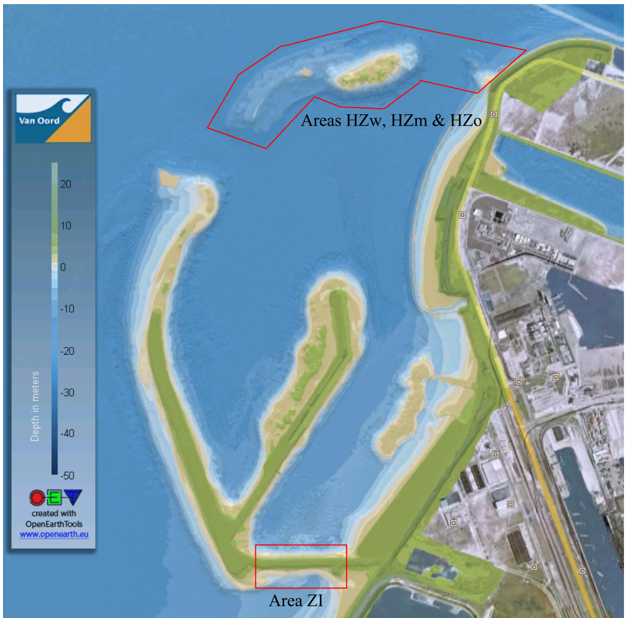
Figure H.12: Overview of the Maasvlakte II project. Survey data of March 2 th , 2010.
