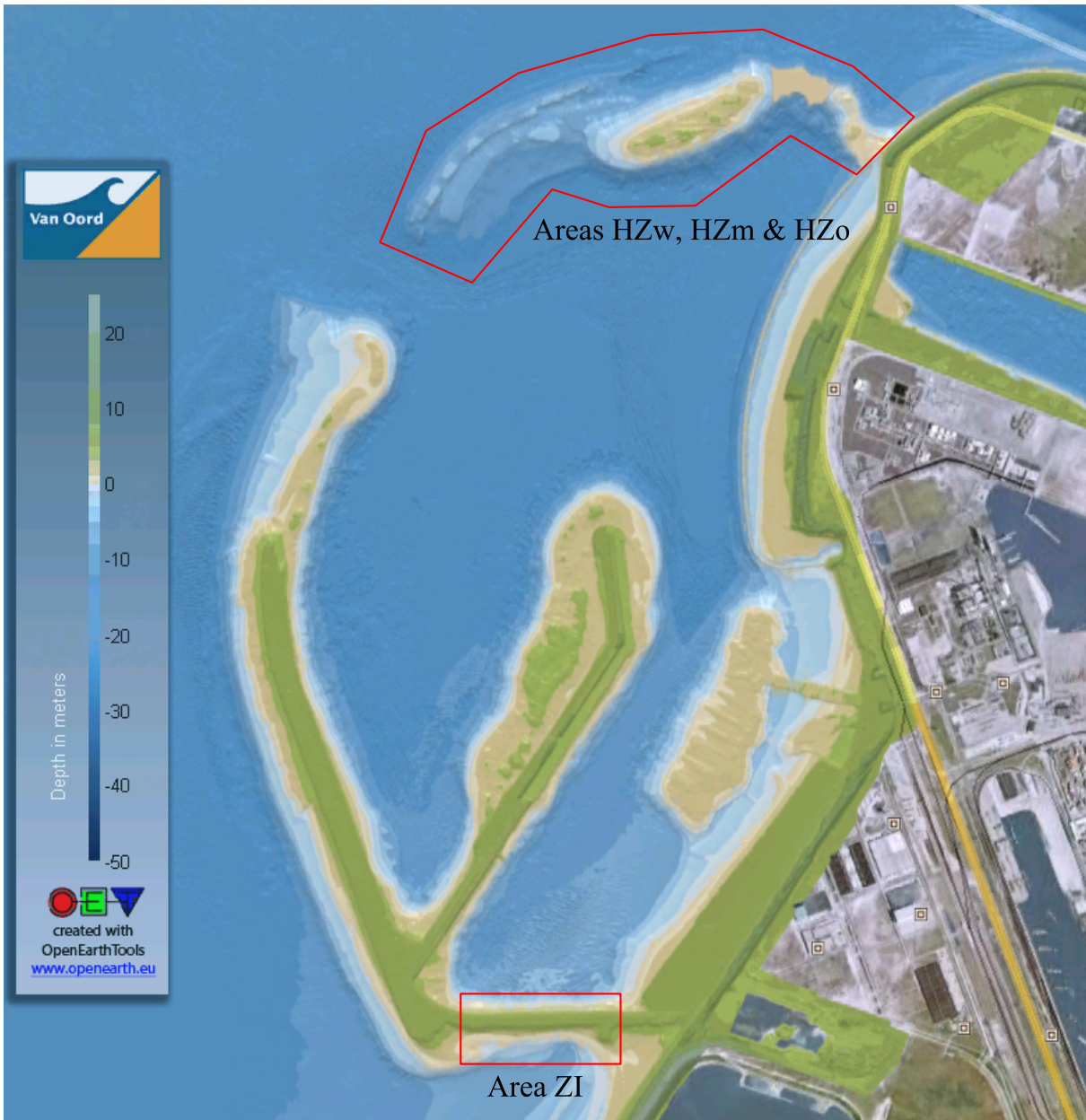
Figure H.13: Overview of the Maasvlakte II project. Survey data of April 2 nd , 2010.
