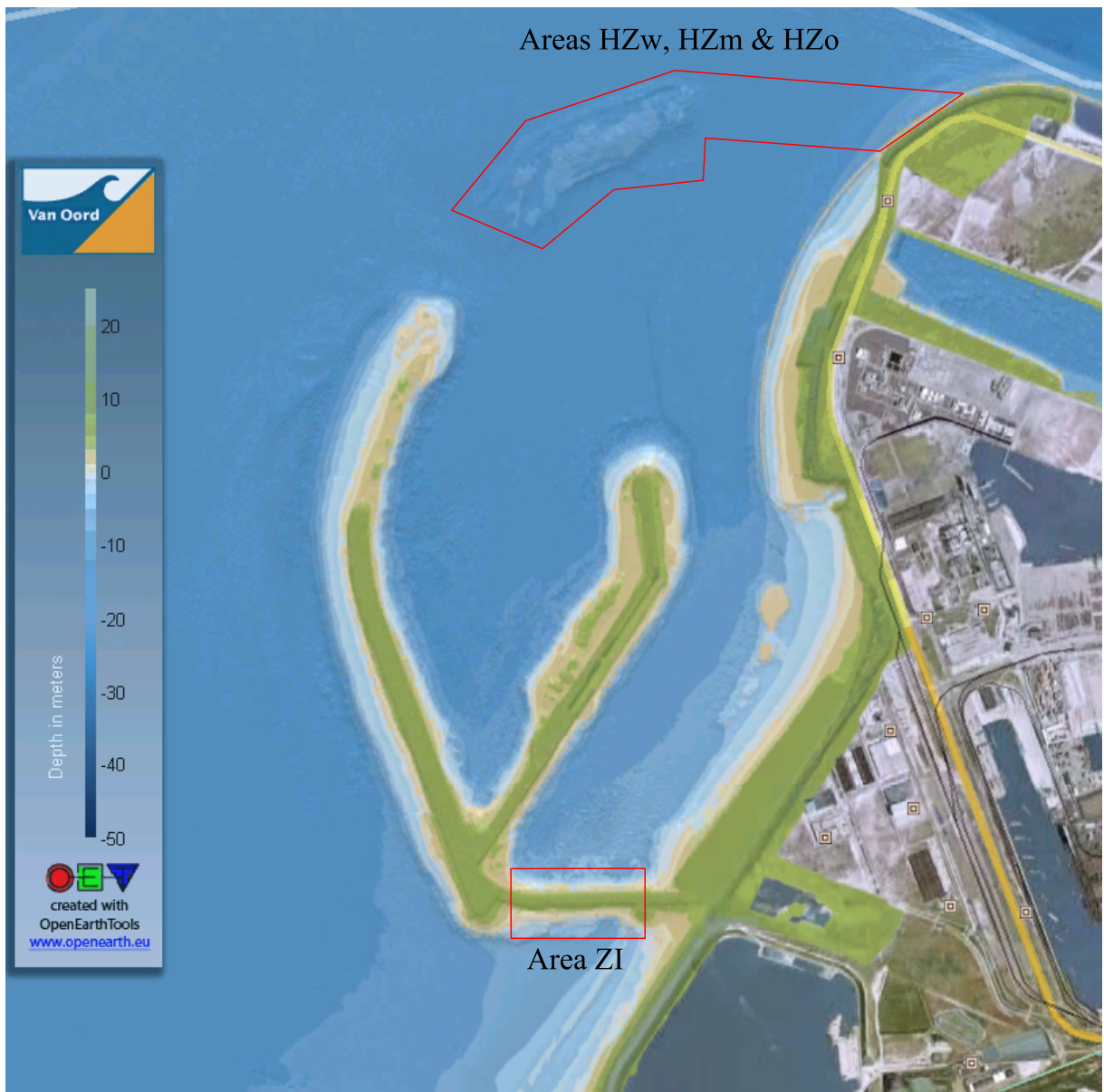
Figure H.10: Overview of the Maasvlakte II project. Survey data of December 30 th , 2009.
