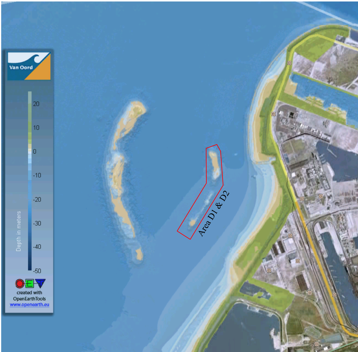
Figure H.3: Overview of the Maasvlakte II project. Survey data of June 2 nd , 2009.
