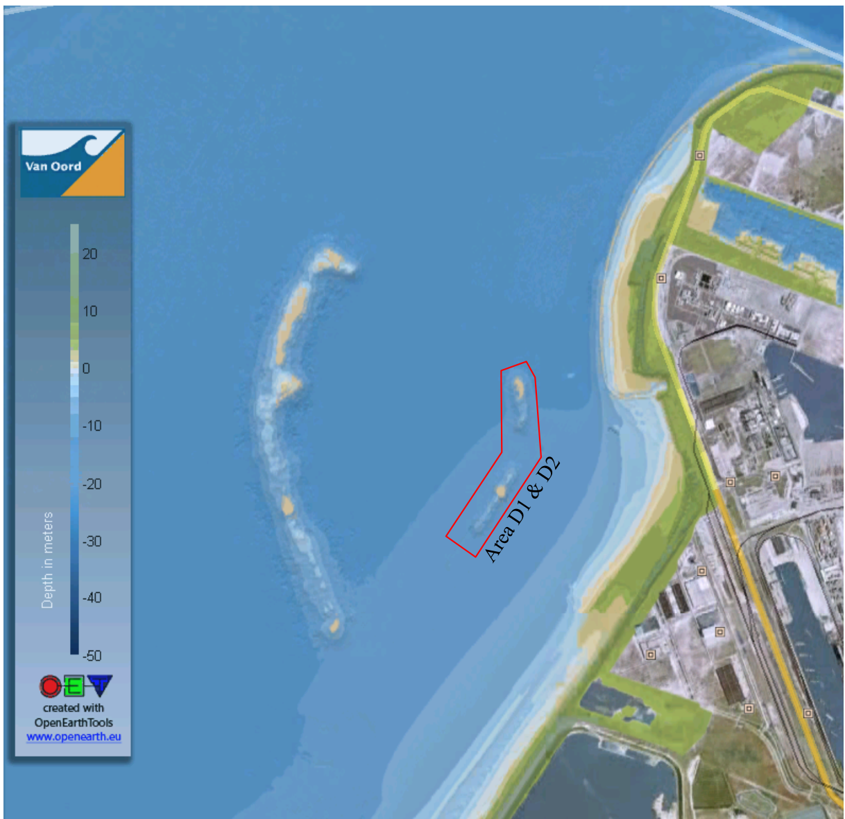
Figure H.2: Overview of the Maasvlakte II project. Survey data of April 29 th , 2009.
