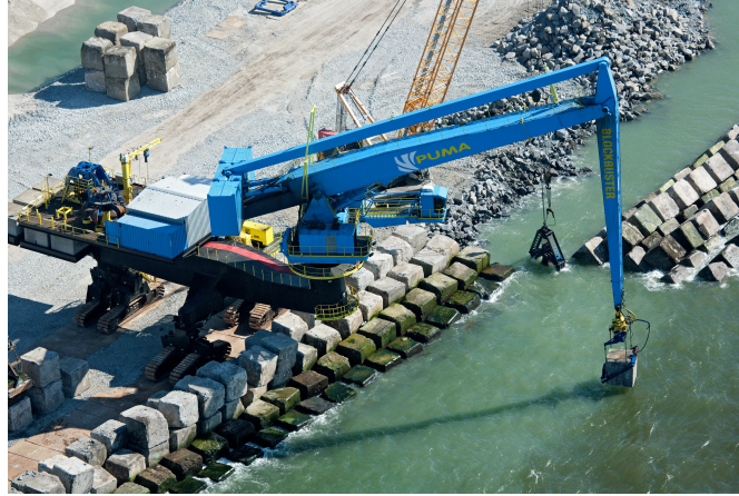
Figure 3.6: “Blockbuster” placing concrete blocks in the hard sea defence. (Courtesy PUMA)
