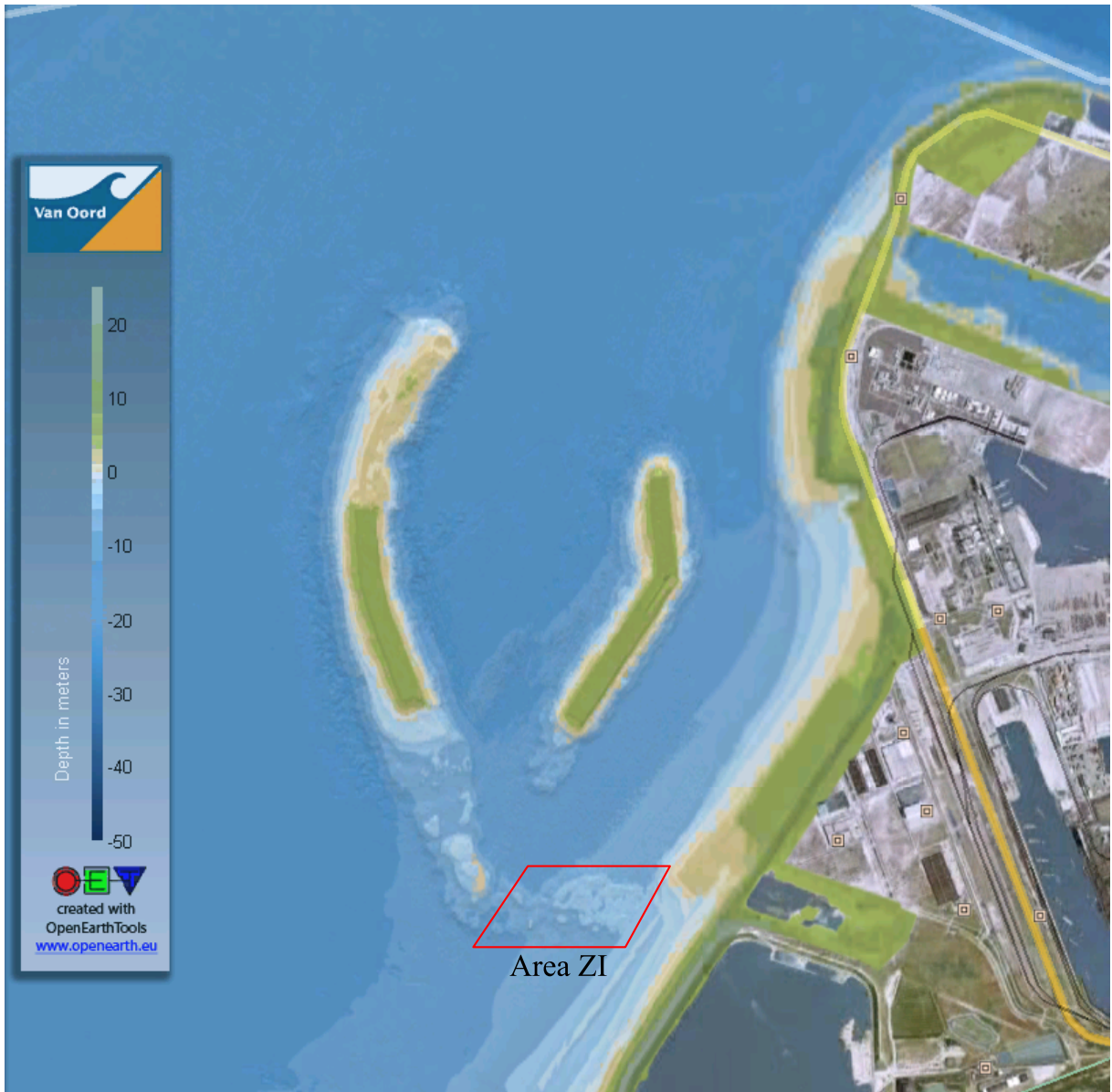
Figure H.6: Overview of the Maasvlakte II project. Survey data of August 30 th , 2009.
