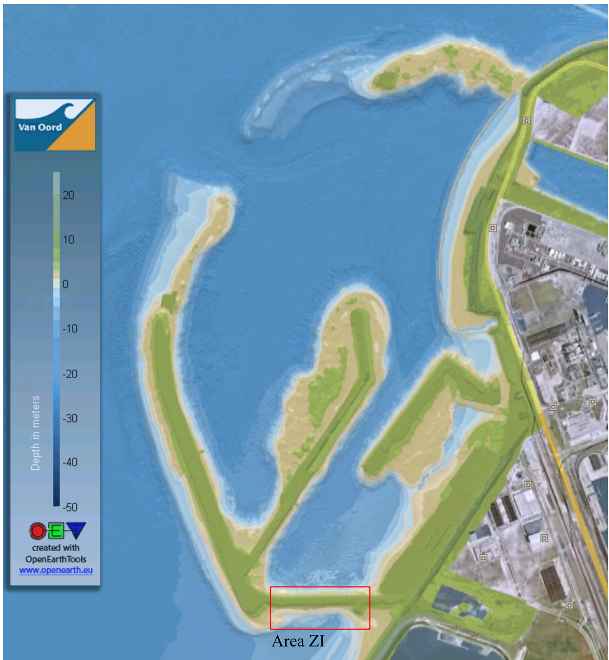
Figure H.14: Overview of the Maasvlakte II project. Survey data of May 1 st , 2010.
