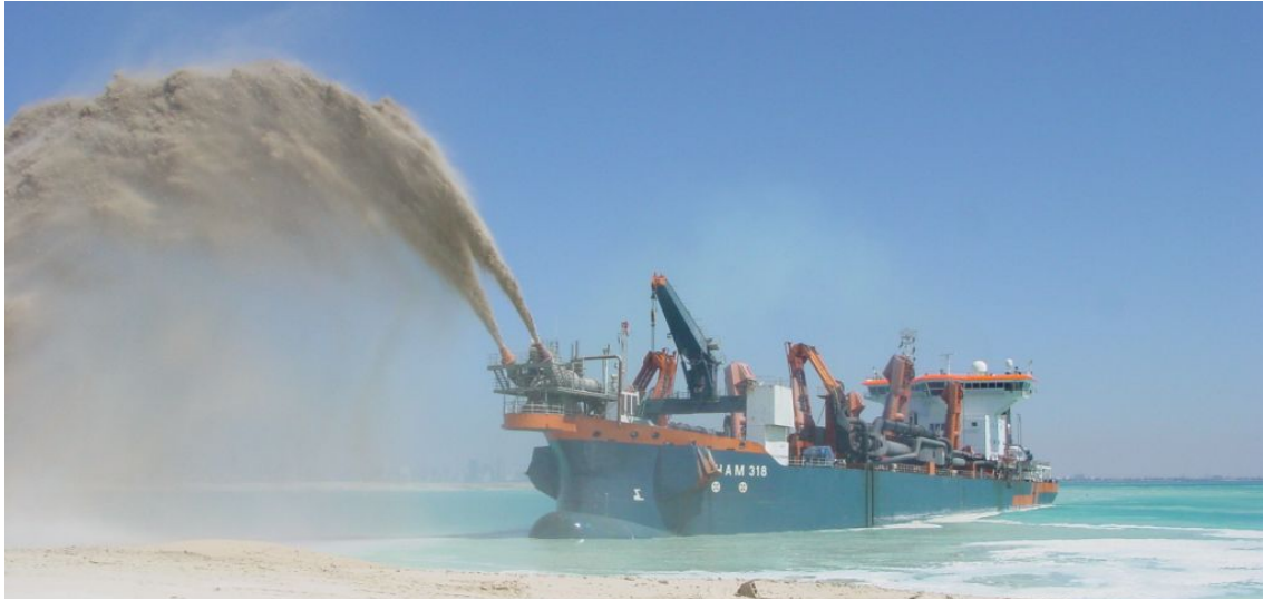
Figure 4.3: TSHD “HAM 318” rainbowing with two nozzles at Palm Deira, Dubai ( Courtesy Van Oord )
