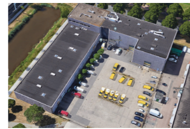
Small distribution centre from DHL in Amsterdam Oost near the city, the perfect location for a UCC
