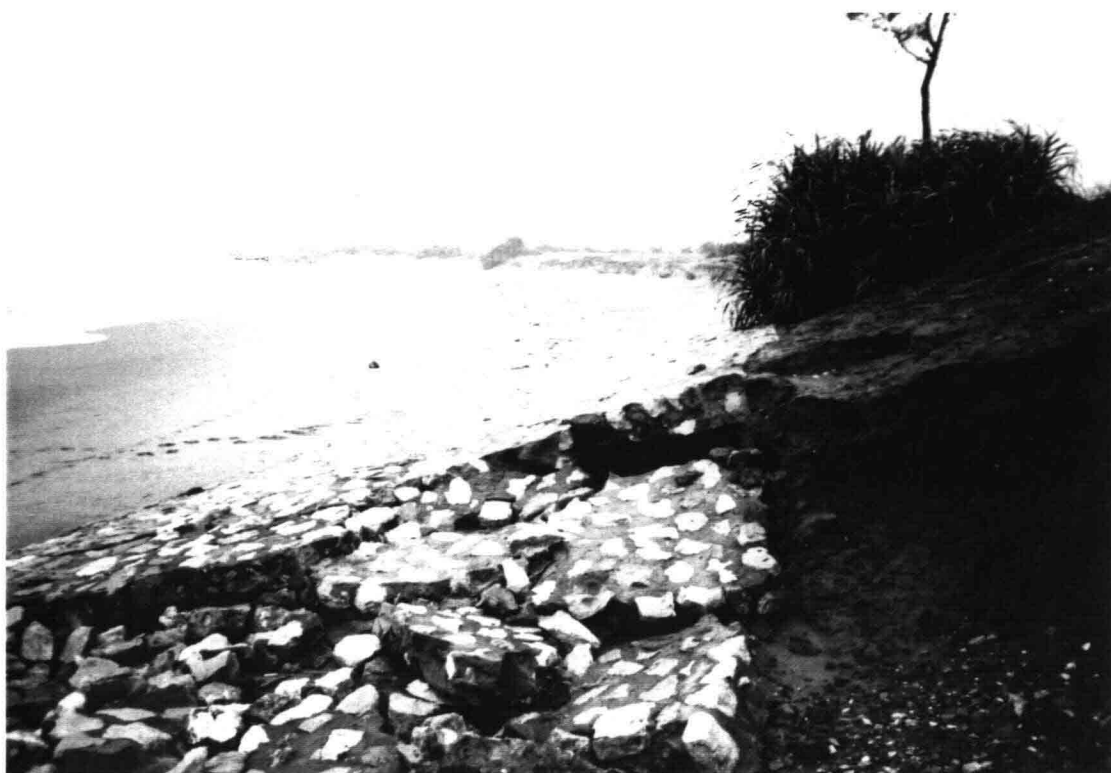
Picture I.4 Damage of concrete grouted stones revetment in Hai Hau District
