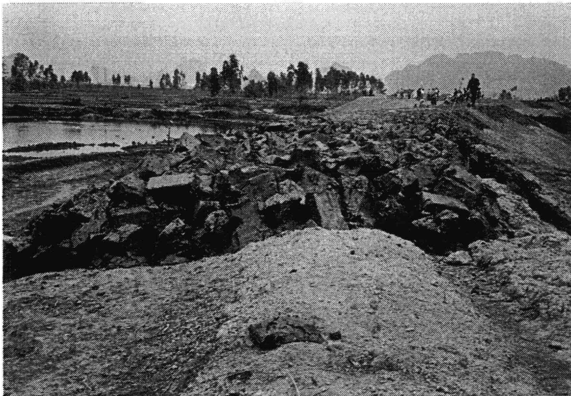
Figure 5.1 Earthfill of clay: difficult to compact
