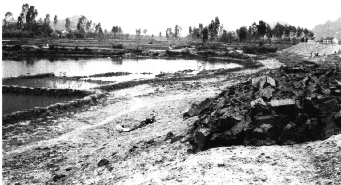
Picture I.3 Excavation close to the inner toe of the dike
