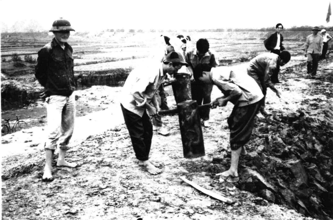
Picture I.9 Dike under construction in Yen Hung District
