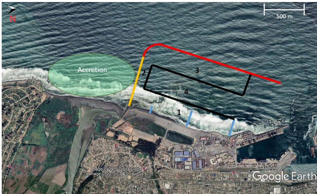
Figure 5.12: Building with Nature construction of the port expansion
