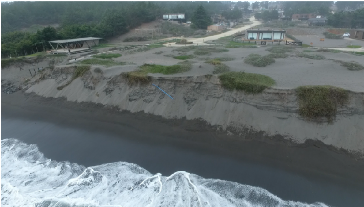
Figure 5.14: Erosion which threatens houses (Recordon, 2018)
