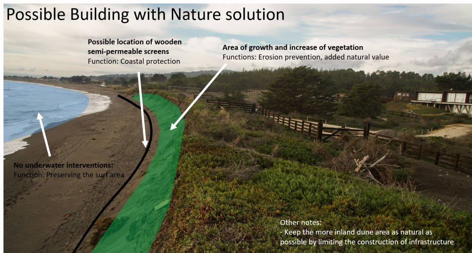
Figure 5.24: Summarizing picture of the possible Building with Nature solution of the beach north of Punta de Lobos
